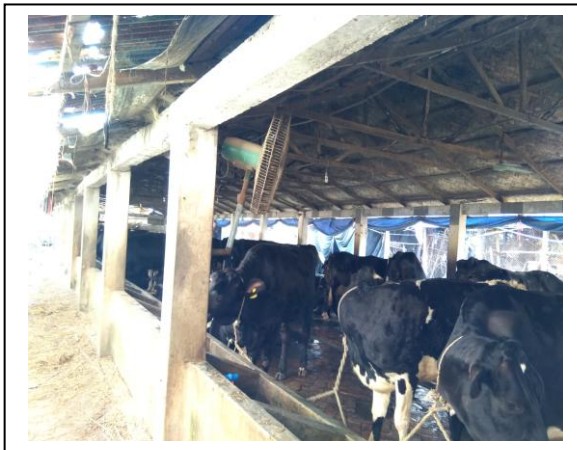
Figure 7: Animal shed of farm C (Low shed height and poor ventilation)
