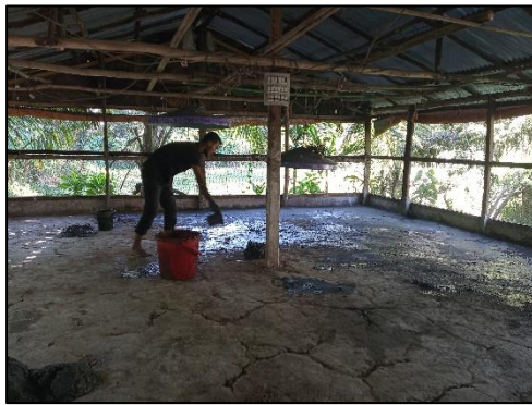
Figure 3.1: Cleaning and disinfection of shed floor. Preparing shed for experiment.
