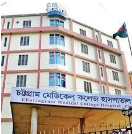
Fig-3.1 Chittagong Medical College Hospital
