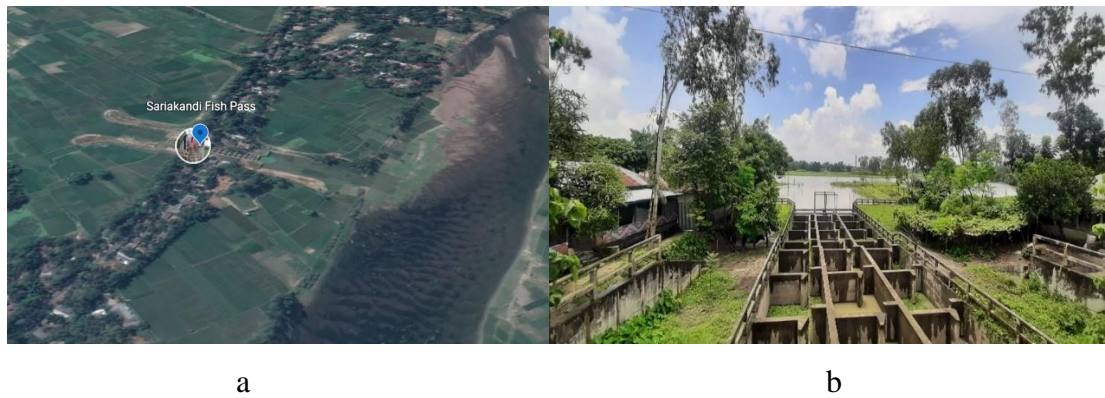
Plate 01: View of the research location: a. Aerial view; b. Vertical slot type fish pass
